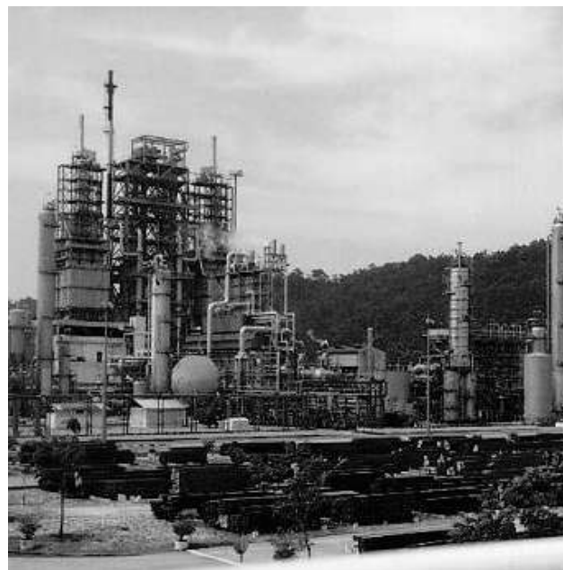
Figure 5. Perwaja Steel Sdn Bhd-HYL Direct Reduction Plant
